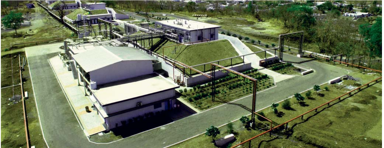
^ Defence Manufacturing Facility
